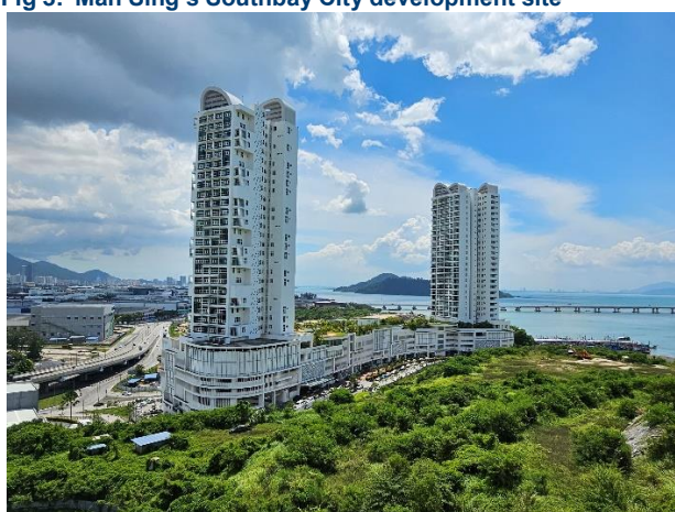
Fig 3: Mah Sing's Southbay City development site
